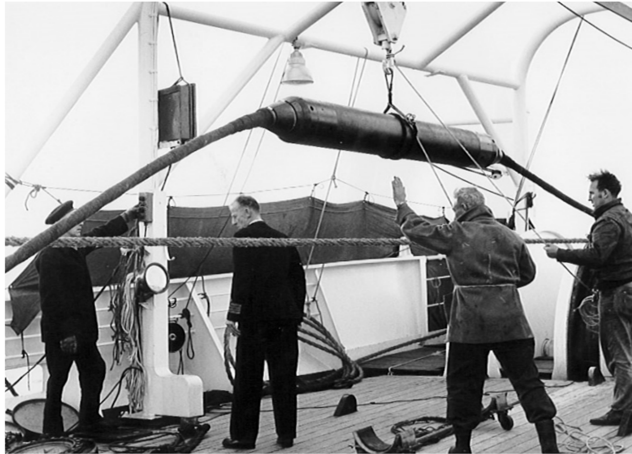
Laying a Rigid Housing Repeater
