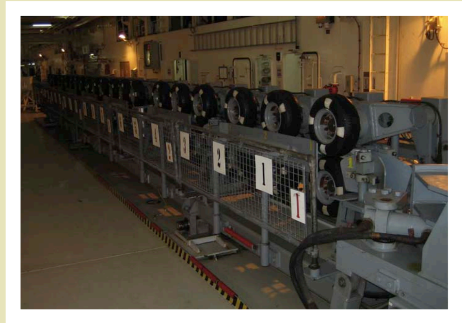
Linear Cable Engine (Courtesy of Alcatel-Lucent)
