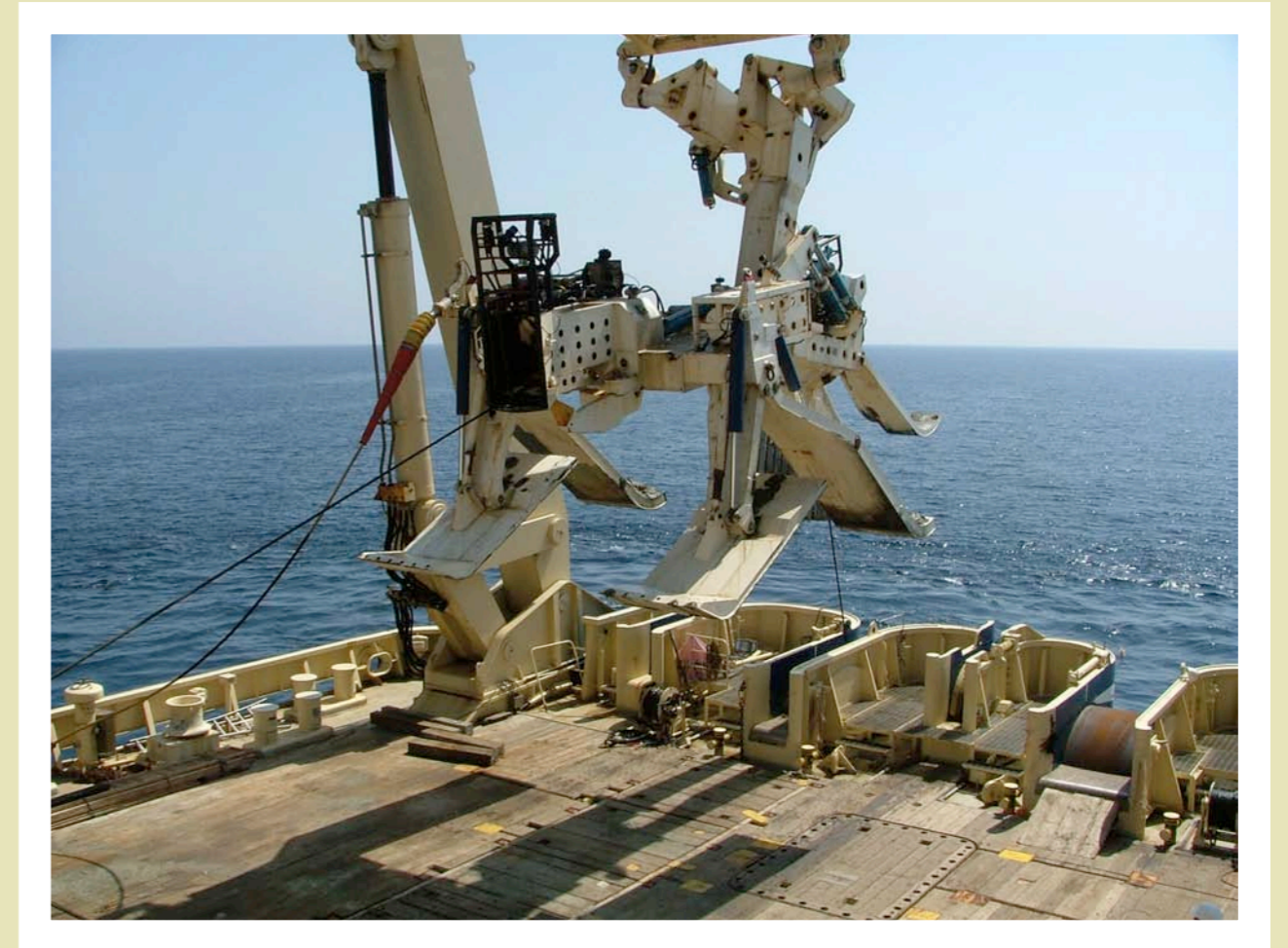
Heavy-Duty Plough Being Deployed
