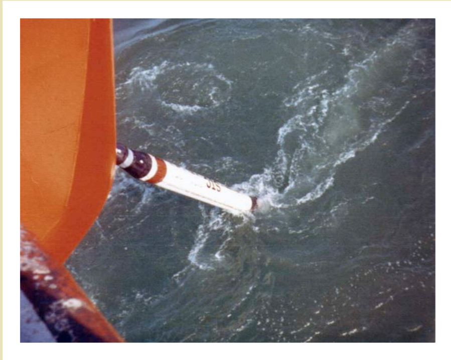
STC Repeater being deployed from C S Alert , 1974
