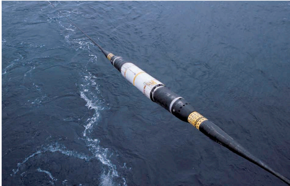
ASN Optical Repeater Being Deployed
